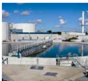
Waste water treatment
